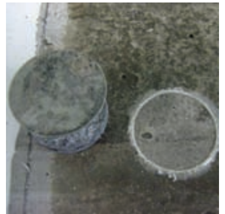
Picture 3 145 psi delamination
