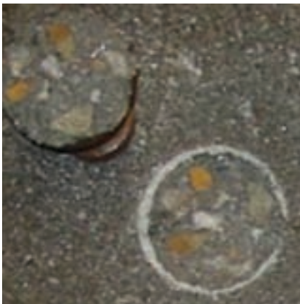
Picture 1 1190 psi concrete failure
